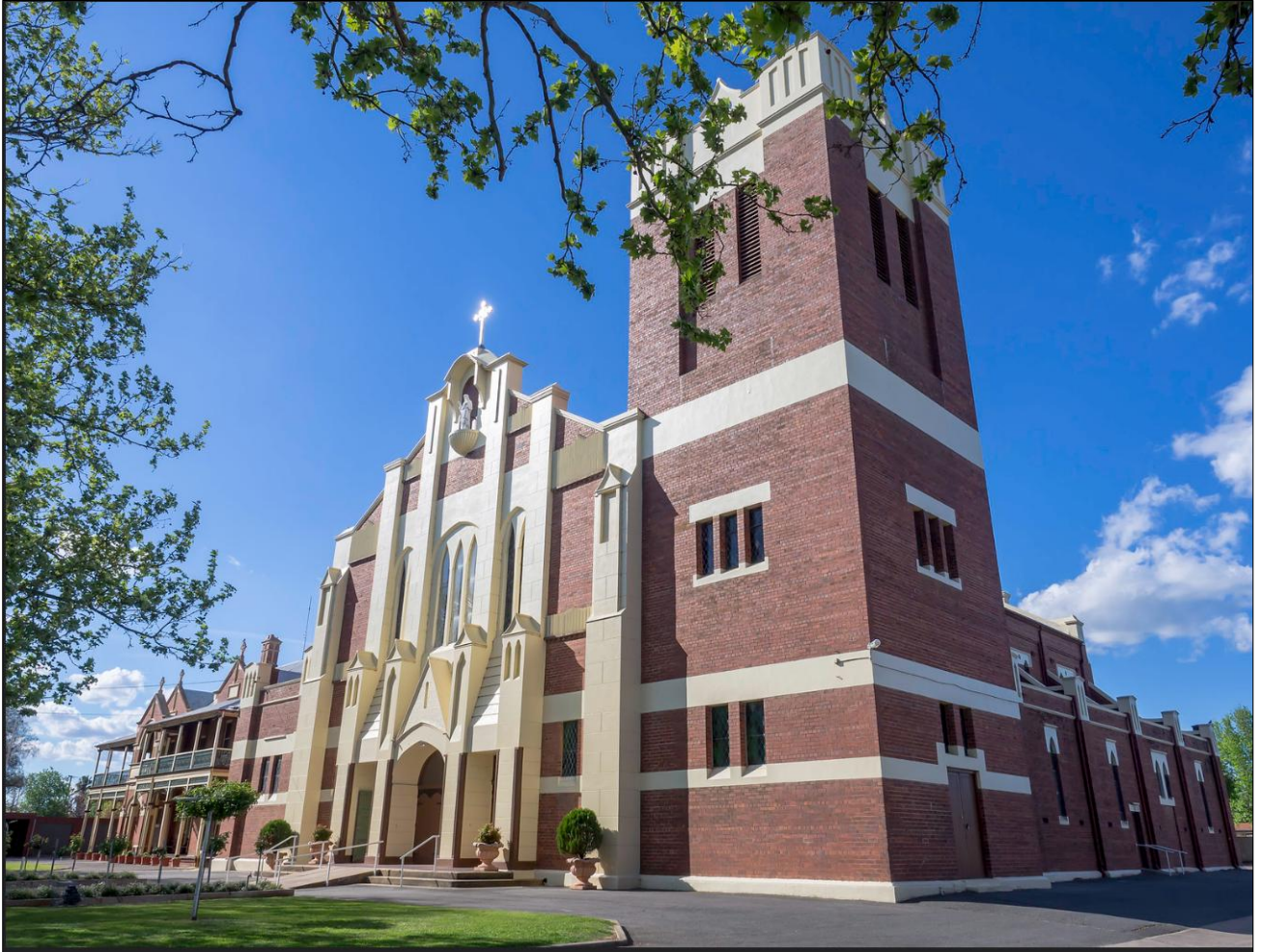
Figure 9 Sacred Heart Church –construction commenced 18 November 1915
