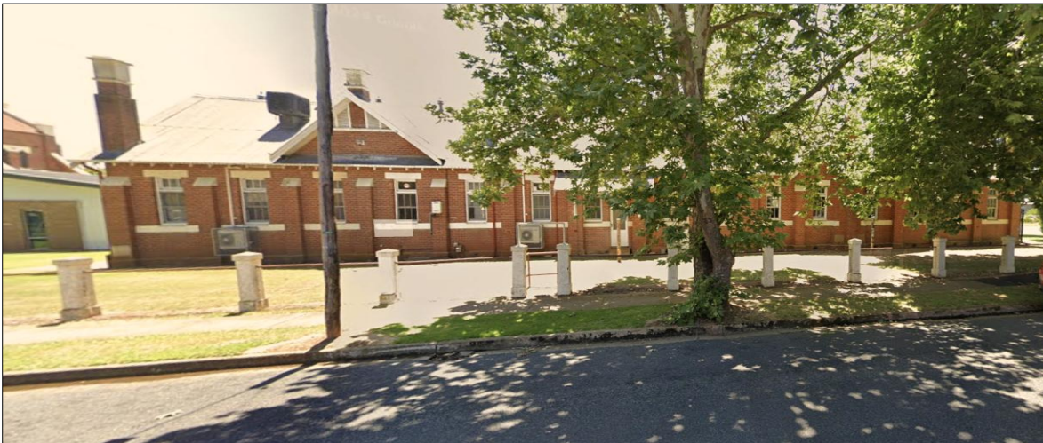
Figure 15 Former De La Salle Brothers School building viewed from Morris St
