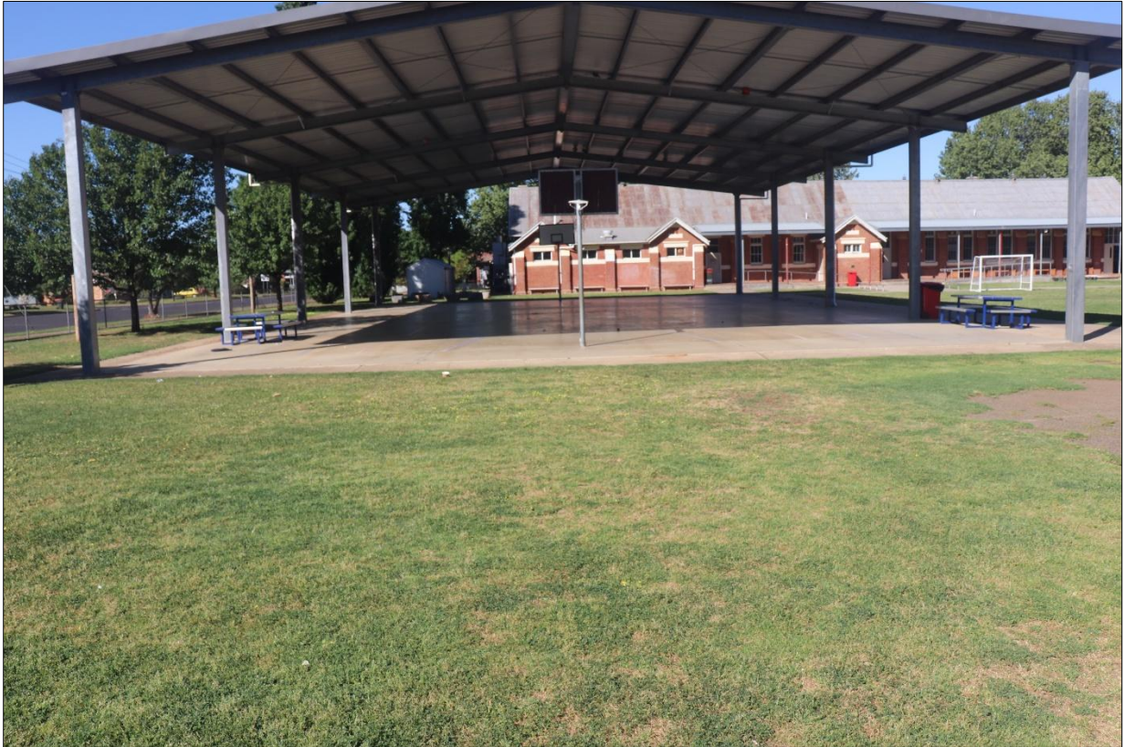
Figure 22 COLA to be demolished
