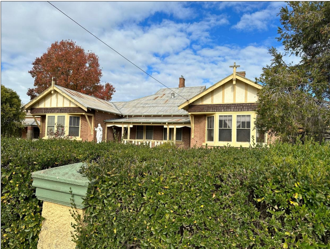
Figure 13 Convent building east of the primary school block
