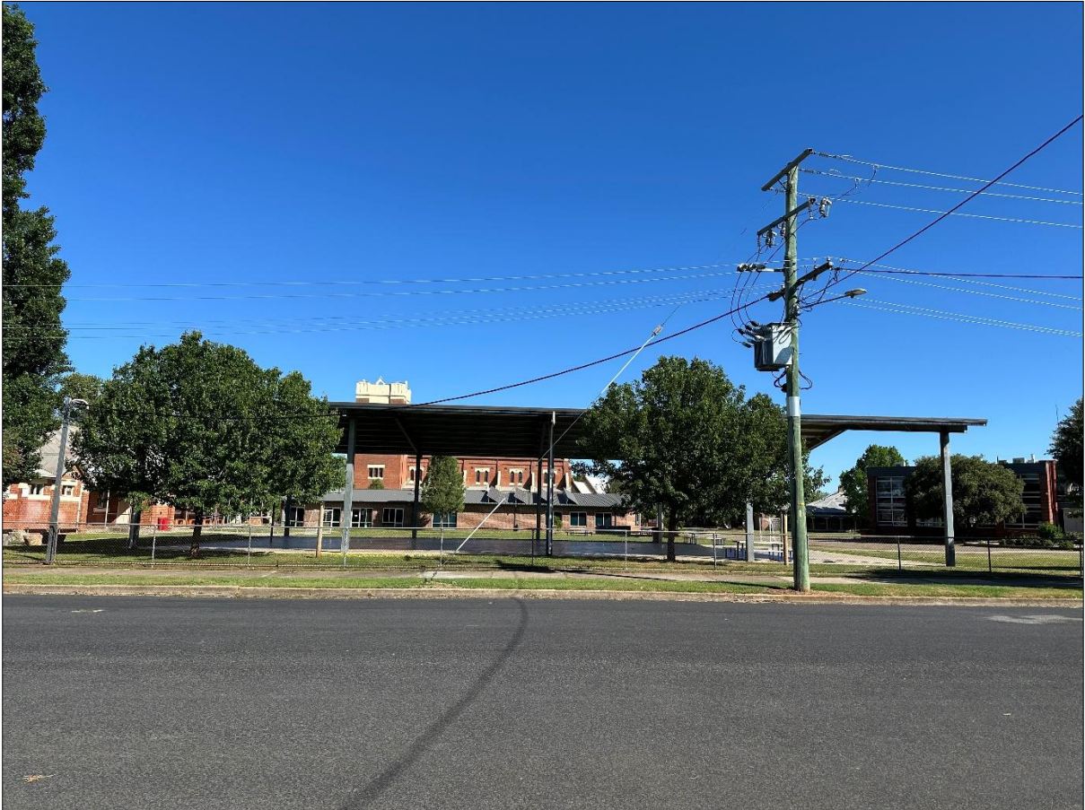
Figure 17 COLA to be demolished
