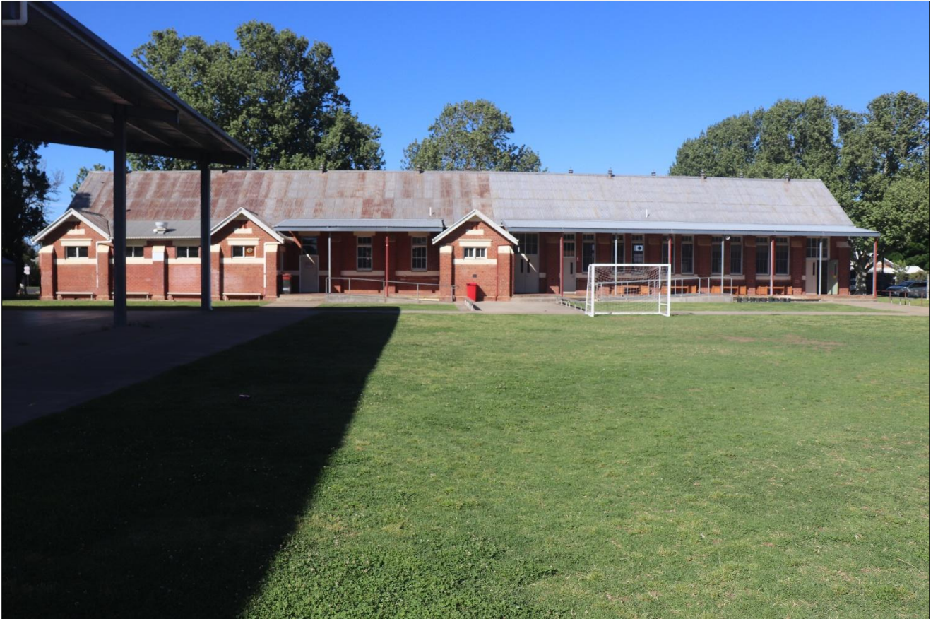
Figure 16 Former De La Salle Brothers building viewed from within site
