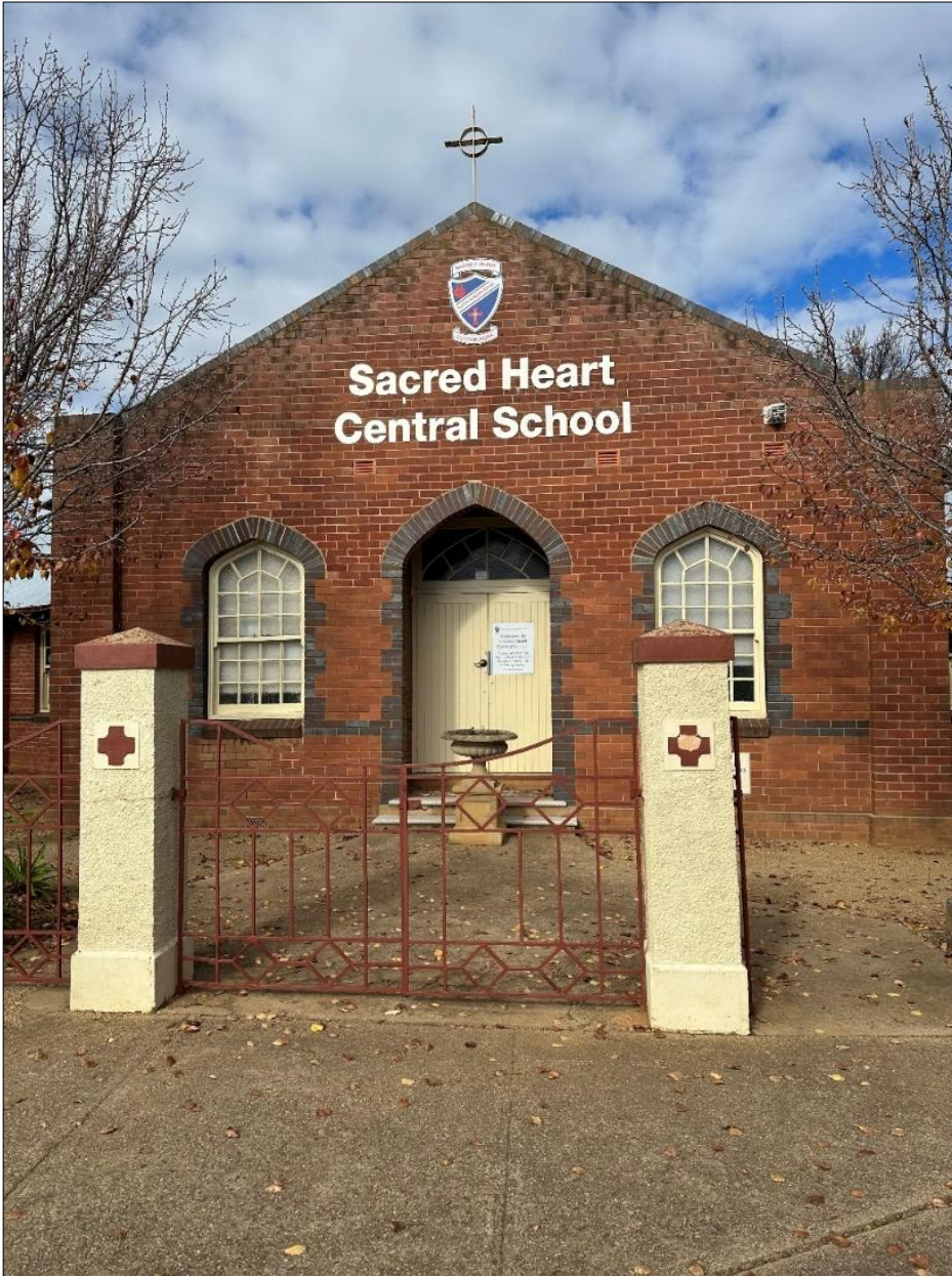
Figure 11 Former external entrance to the primary school
